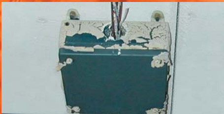
Cable junction boxes with connected cables after testing
