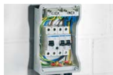
British Standard installation with earthed armored cables
