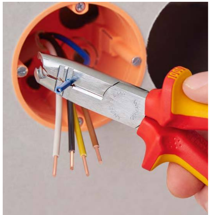
Cutting when shortening single conductors
