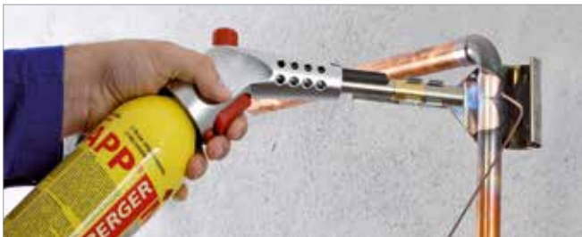
Brazing in gas installation
