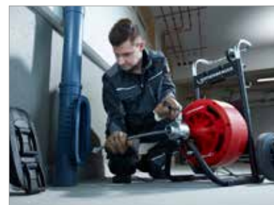
Cleaning of a down pipe with 16 mm spiral
