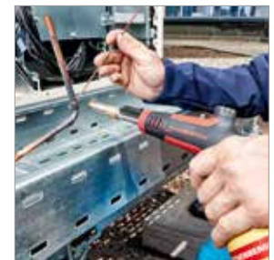
Brazing in refrigeration / air-conditioning technology
