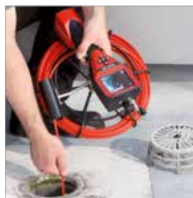
Inspection of rain downpipes
