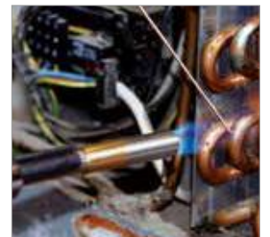
Brazing in refrigeration / air-conditioning technology
