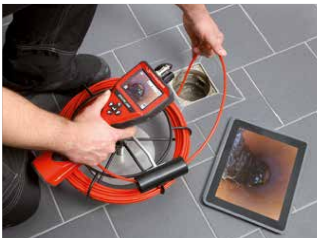
Inspection of basin drains
