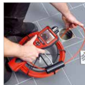
Inspection of floor drains
