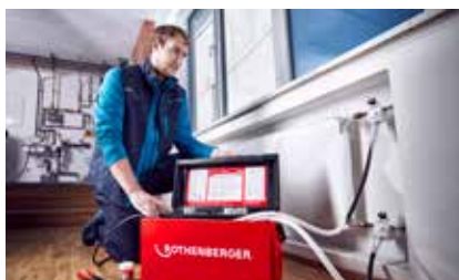
The freezing process starts automatically after installing the freezing clamps
