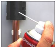
Inject spray into clamp
