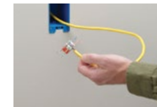
2. Determine wiring scheme. Dress all four pairs (eight wires).
