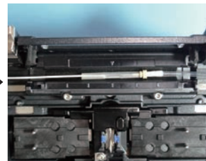
3. protection sleeve shrinking
