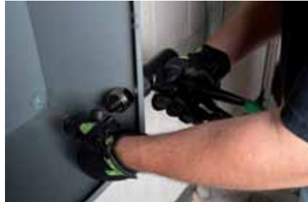
Fix the die and start punching.
