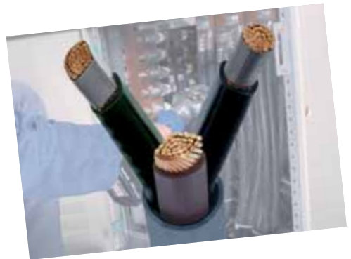
Round-crimping sector sleeves in three steps.
