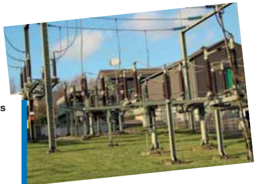
Aluminum compression cable lugs are frequently used in power distribution.
