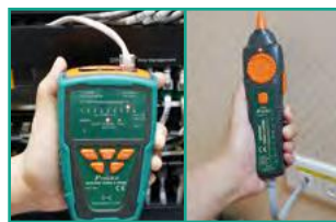
Verify LAN/ telephone cable condition
