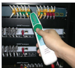
Copper cabling detecting
